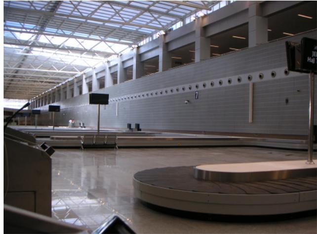
IC16 (Iconyx array): thin, small and hardly to be recognized
